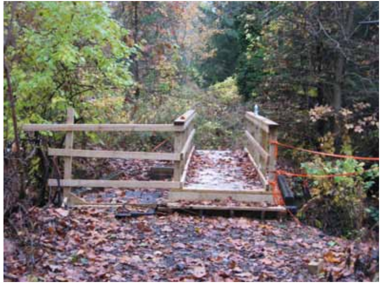
Bridge over Green Tree Run
