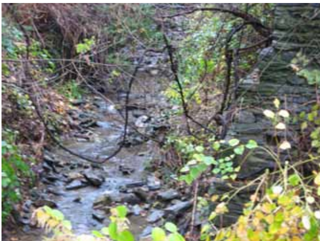
Retaining wall by stream
